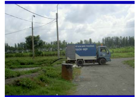
Discharge of septage into a dump located in Hau Giang province
